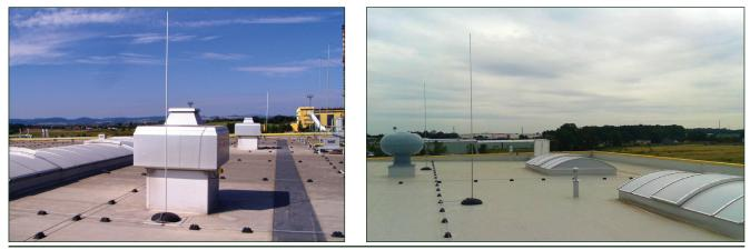
Figure AT:3 - Free-standing Air Terminals installed with 8mm diameter aluminium conductor
